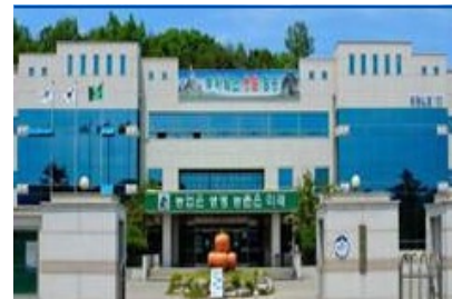
Gyeongsangbuk-do Technical Center for Agricultural Cooperative _ IOR-80A
