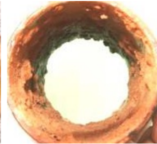
3rd inspection (May 6, 2009)
