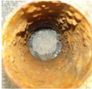
1st inspection (January 29, 2008)
