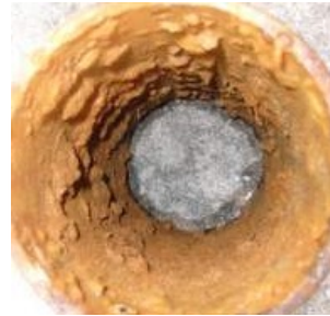
2nd inspection (July 25, 2008)
